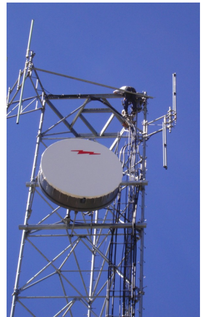
Tower Climbers replacing the dual-band antenna with separate VHF and UHF antennas
