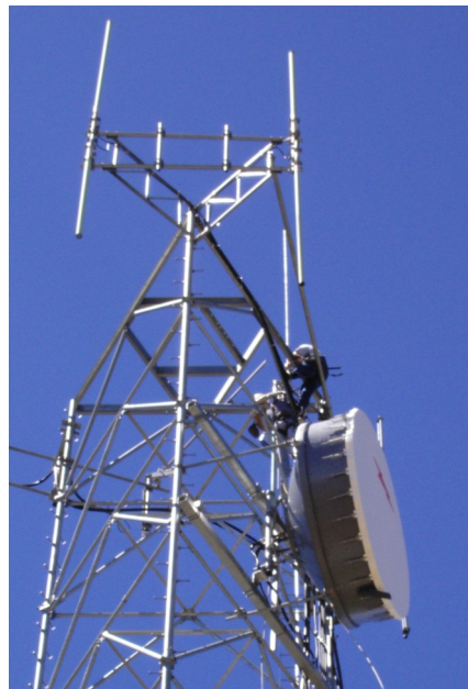
Tower Climbers replacing the dual-band antenna with separate VHF and UHF antennas
